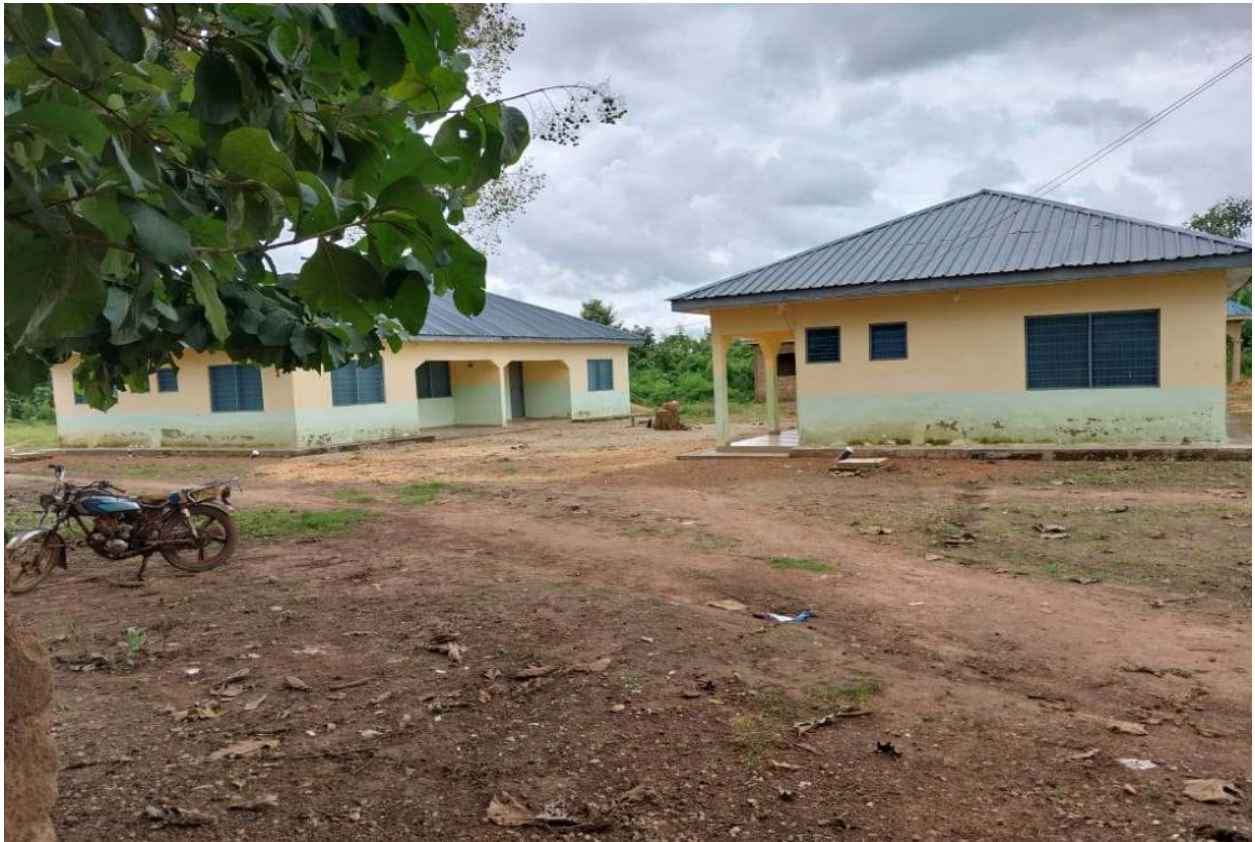
FINAL PAYMENT A CHPS COMPOUND COMPLETED AT ABUNYANYA
