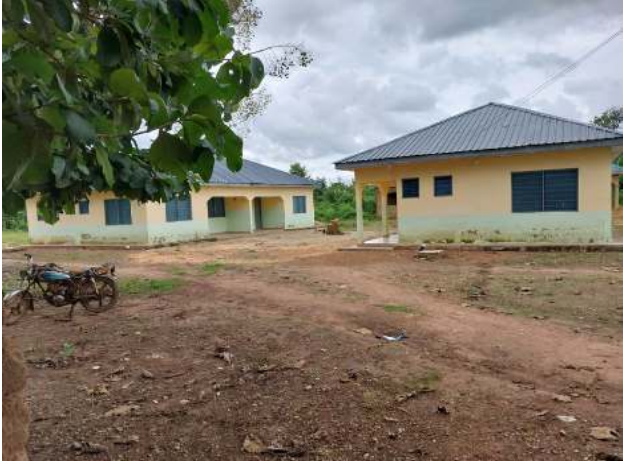
1No. CHPS CPOMPOUND WITH STAFF QUARTERS COMPLETED AT ABUNYANYA
