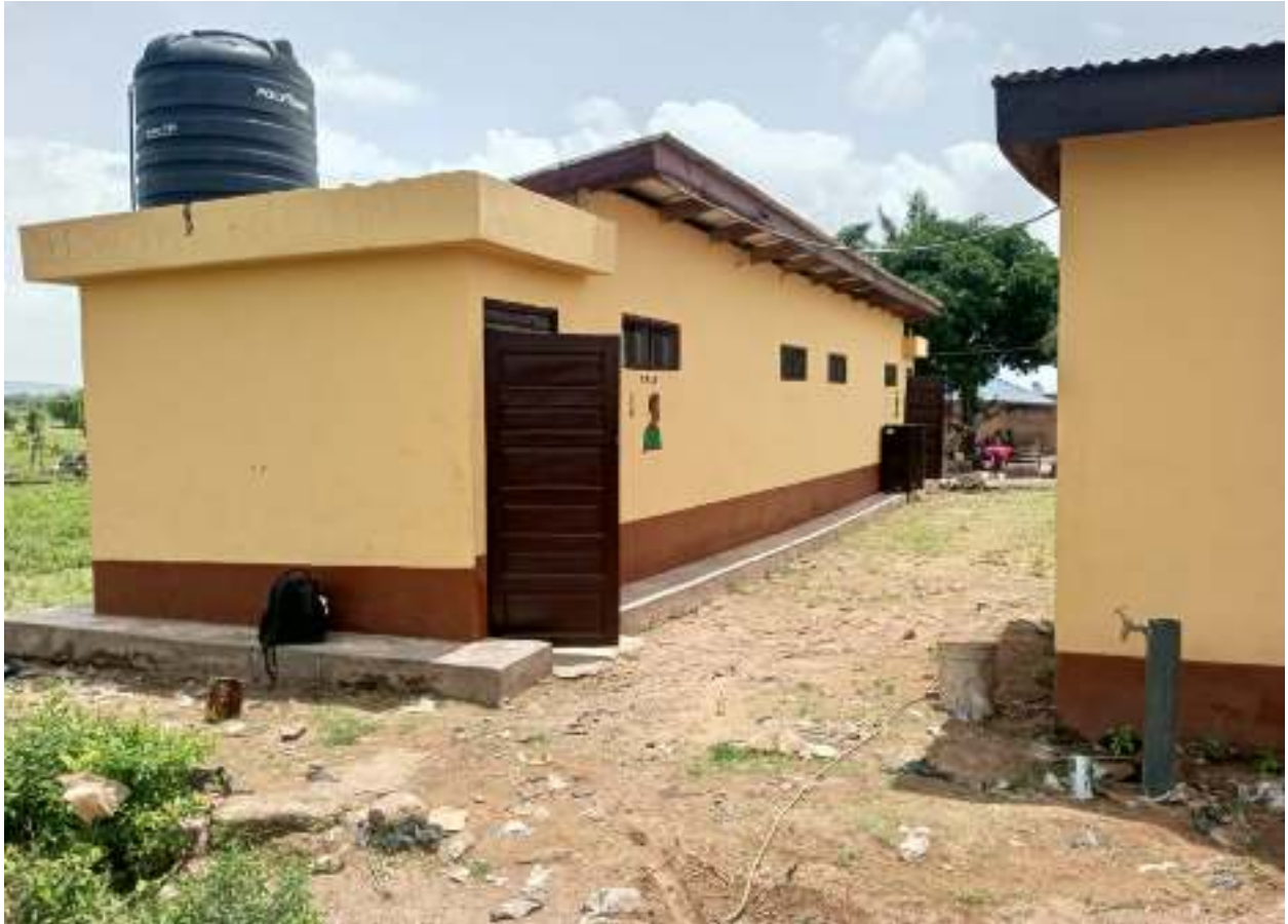
COMPLETION OF 1NO. 10SEATER W/C AT DAMANKO YAM MARKET
