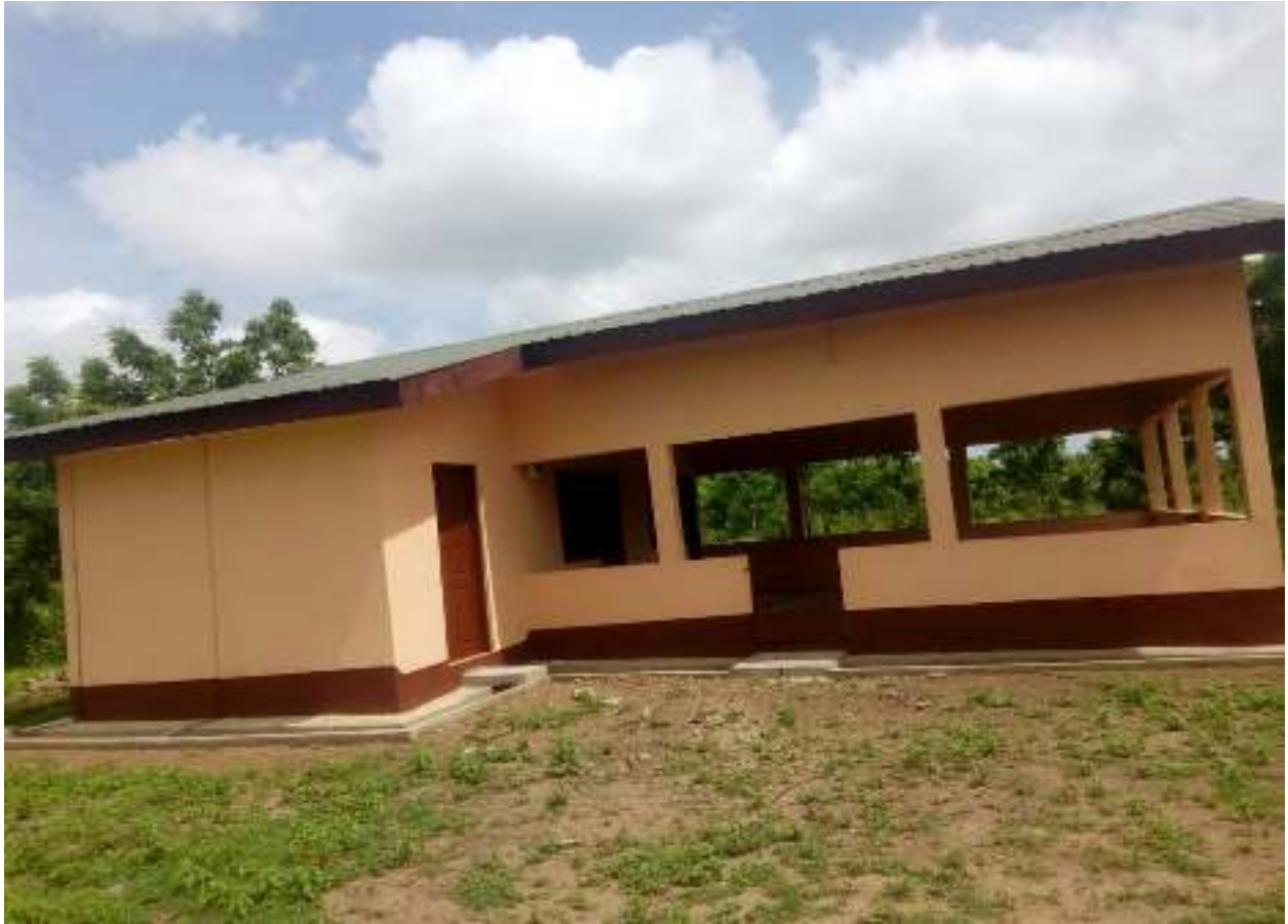
1No. CHPS CPOMPOUND WITH STAFF QUARTERS COMPLETED AT OBUNJA
